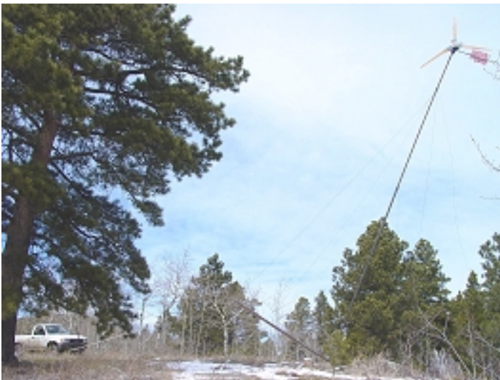
A 40-foot tilt-up tower being raised via pickup truck and gin pole. Colorado, USA
